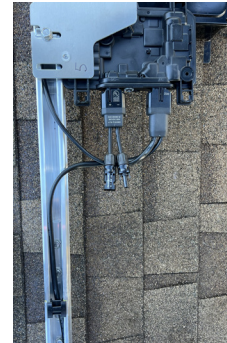
Wire management clip installed on the roof
