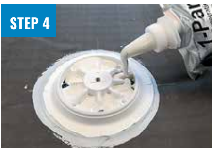
FILL WITH CHEMLINK 1-PART & PLACE CAP
