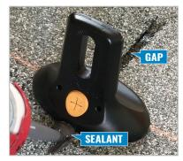
NOTE: When **FLASH**LOC is installed over gap between shingle tabs or vertical joints, fill gap/joint with sealant between mount and upslope edge of shingle course.
