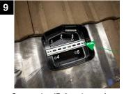
Secure the JB-2 to the roof decking using (5) #10 x 1-1/4" Phillips pan head screws (provided). Install outdoor-rated, UL 514B, NEMA 3R approved fittings and/or strain reliefs to the EAST, WEST and SOUTH side walls of JB-2 and complete wiring installation. Up to 1" raintight fittings are all acceptable. Clean off all burs.
