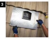
Insert aluminum flashing with the top edge underneath the row of tiles above, center pentagon flashing in opening.
