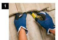
Determine location for JB-2 on the roof surface. Loosen tiles in the row above desired location. Remove the roof tile(s) where the JB-2 will be located.
