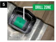
Place the JB-2 base into the opening in the flashing. Using a drill bit, drill through the box & roof simultaneously within the approved 'Drill Zone'. Verify penetration hole(s) are on either side of a rafter but not over or through a rafter/truss.
