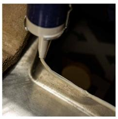
Within the Drill Zone, add the appropriately sized hole(s) into the attic. Apply generous sealant to the underside following the sealant guide. Also apply sealant to sidewalls of the raised portion of flashing. Install fittings and connectors as needed. After connections are complete, finish by installing lid. Hand tighten until screw head fits snug on lid.
