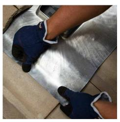
Determine location for the JB-2 on the roof. Remove tile, insert aluminum flashing, center pentagon flashing in opening. Press firmly with both hands to form the flashing to the contour of the roof tiles.
